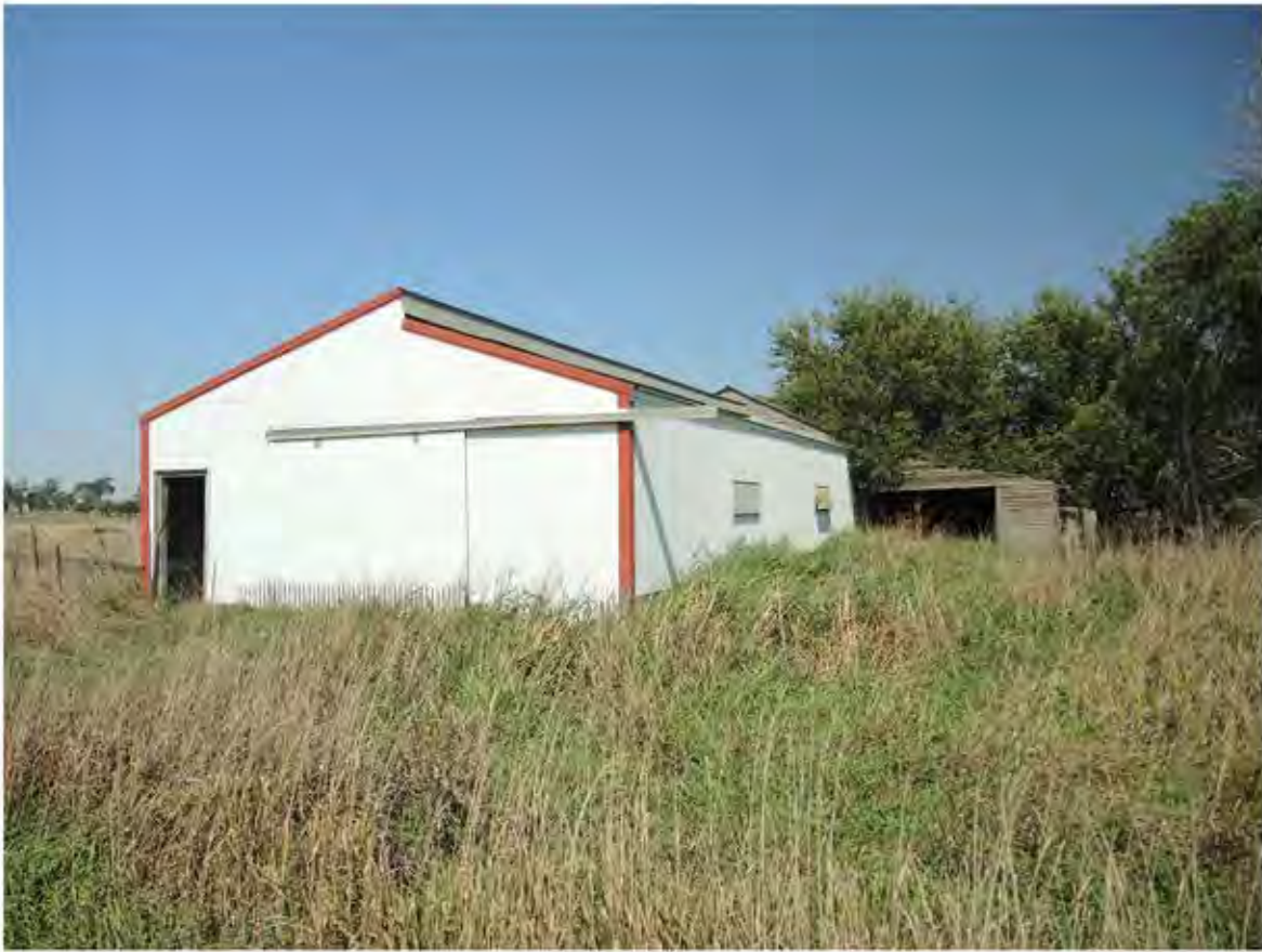
Property includes a 24' X 56' pole shed with steel siding and cement floor.
